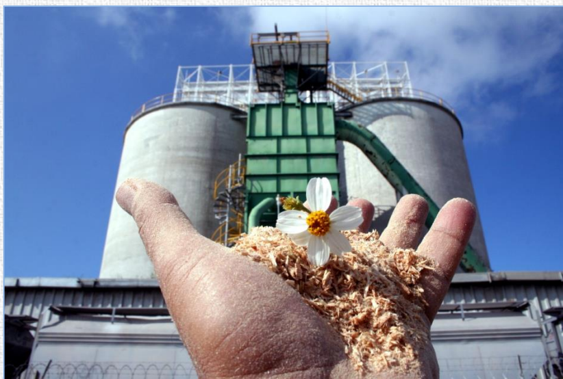
Victor Casillas Romo, CDM project 8035: CEMEX Mexico biomass project at Huichapan cement plant
