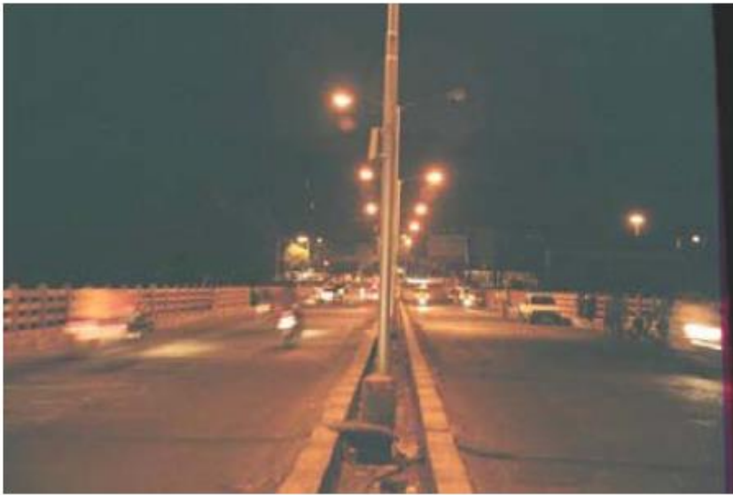
Baseline sodium vapor lights
