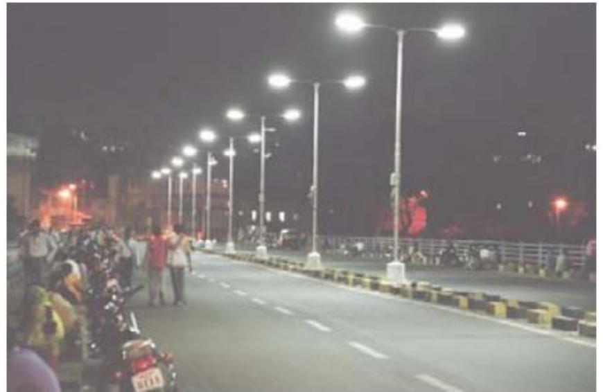
Project T5 lights
