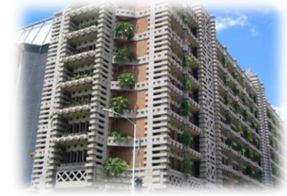
Eastgate: Sustainable building in Harare.
