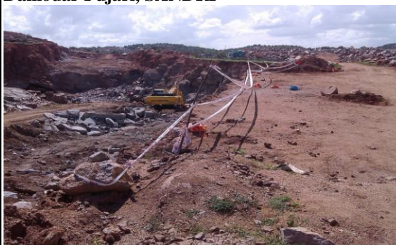
Above: Extensive blasting at the dam site now on going. Photo: Damodar Pujari, SANDRP
