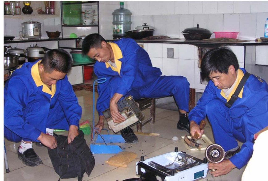
Fitting a Biogas Cooker (Hubei Eco-Farming Biogas Project)
