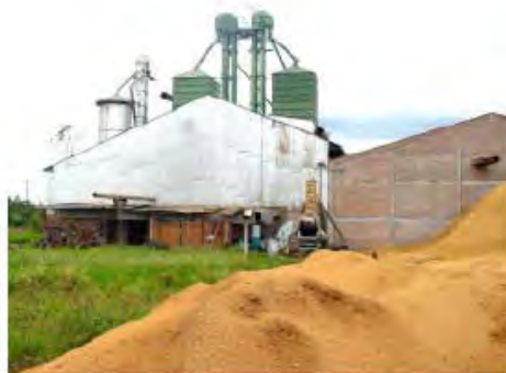
Oven to dryers connection in Bolivian rice mill
