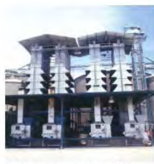
Drying ovens in Costa Rica
