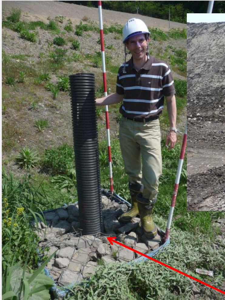
Vertical gas venting wells
