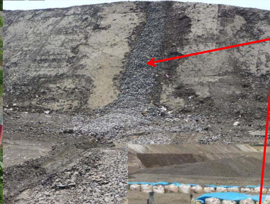
Vertical gravel layers
