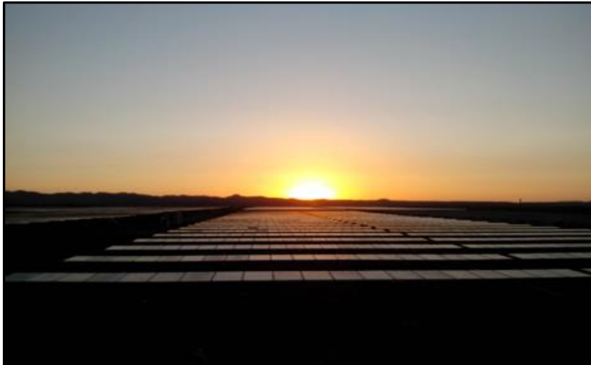
PHOTOGRAPHER: Ignacio Fuertes CDM PROJECT: 7596: Programme for the promotion and development of grid-connected solar PV projects in Latin America COUNTRY: Chile
