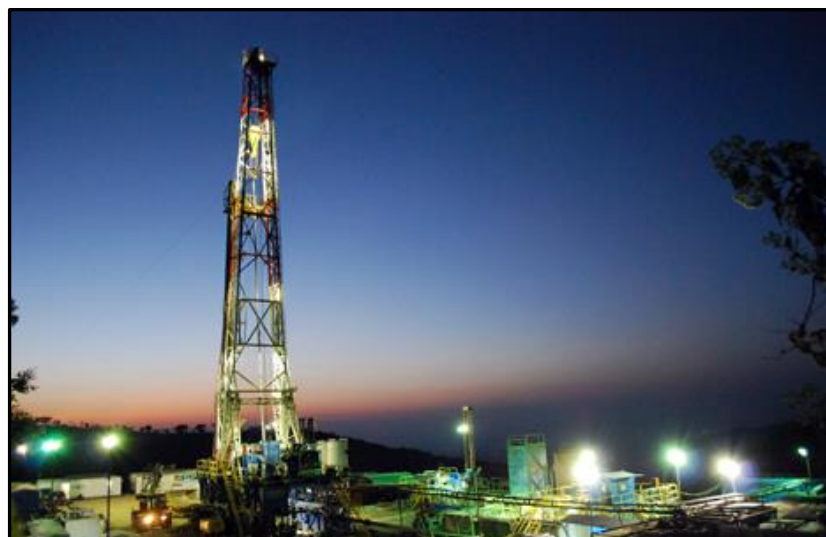
PHOTOGRAPHER: Mauricio Grande CDM PROJECT: 1218: Berlin Binary Cycle power plant COUNTRY: El Salvador
