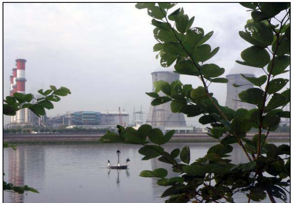
PHOTOGRAPHER: M K Nandi TITLE: A Power Plant With a Difference CDM PROJECT: 1116 1147.5 MW Natural Gas Based Grid Connected Combined Cycle Power Generation Project COUNTRY: India
