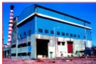
Side view of TG building and transformers
