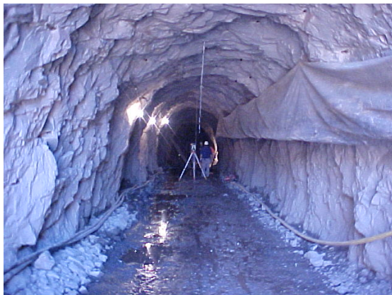
Figure – Cooperluz water tunnel
