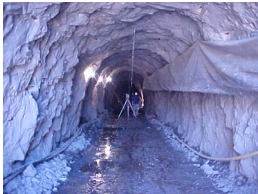
Figure – Cooperluz water tunnel
