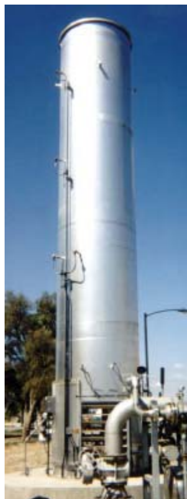
Figure 13. Enclosed Flare installed (source: John Zink, accessed on January 31 st , 2006)
