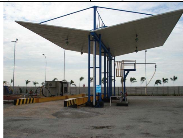
d) LPG loading bay and weighbridge at Odira
