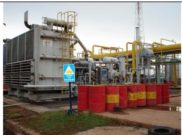
h) Main compressor, gas fired, with barrels of lubricating oil – this is sent for recycling rather than consumed by the compressor
