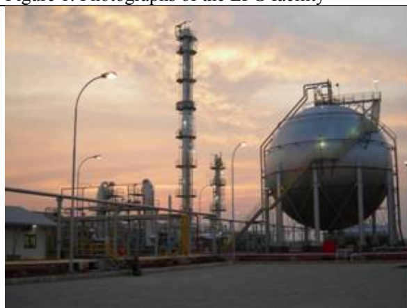
a) Tambun LPG Tank and distillation columns
