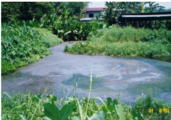
Figure 3 Typical Unlined Anaerobic Lagoons in Swine Farms in Malaysia
