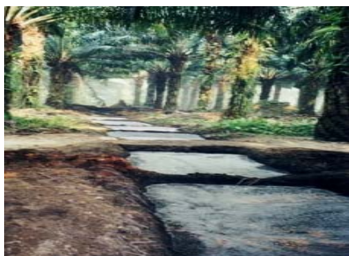
Figure 4 Typical Anaerobic Ponds for Treating POME
