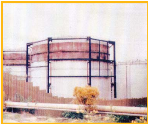
Plate 1 : Floating roof closed tank anaerobic digesters for POME biogas capture at Keck Seng
