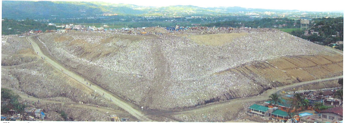
Figure 3 – Payatas disposal site before (up) and after (below) the conversion to a controlled dumpsite
