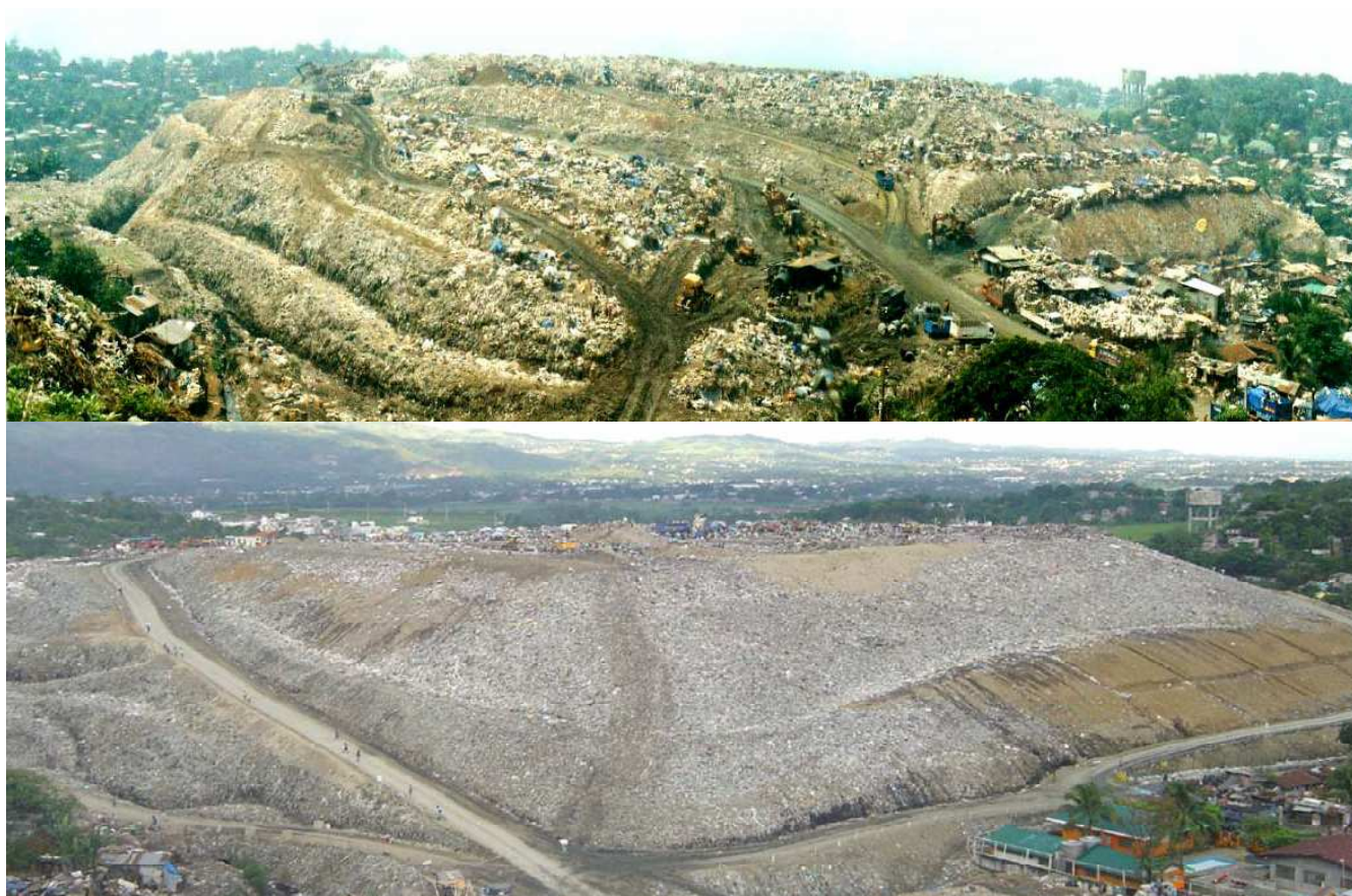
Figure 4 - Payatas disposal site before (up) and after (below) the conversion to a controlled dumpsite
