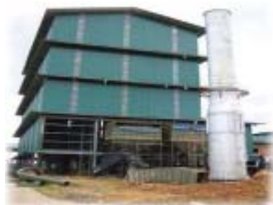
The TSH Bio-Energy Cogeneration plant
