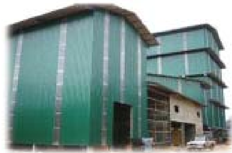
The TSH Bio-Energy cogeneration plant
