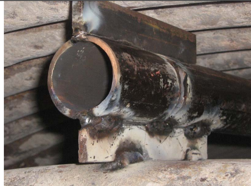
Figure 16: Soot blower repaired
