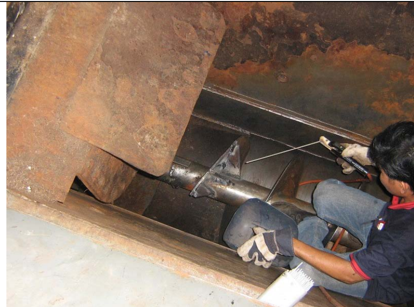
Figure 10: Repair of one of the components of feeding system (screw conveyor)
