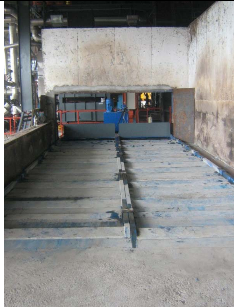
Figure 12: Replacement of new moving due to old one worn out beyond repair
