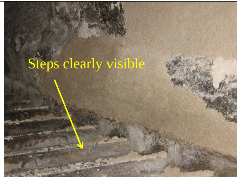
Figure 6: Without clinker, steps of the furnace floor is clearly
