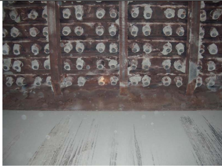
Figure 3: Cyclones cleaned - unblocked
