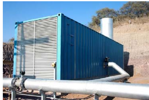
Figure 1.5 Flow meter, inlet gas to flare
