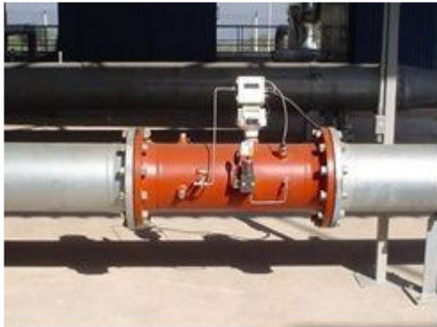
Figure 1.4. Turbine Flow-meter
