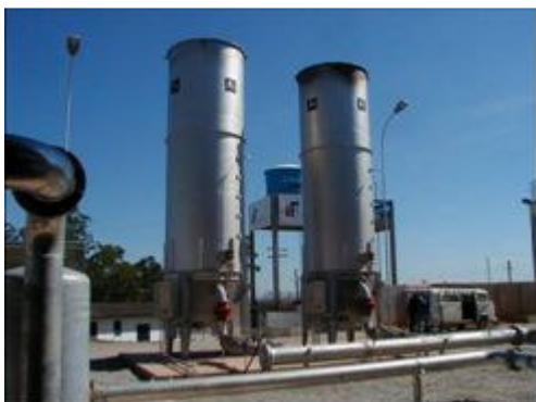
Figure 1.6. Flare used to destroy the surplus gas collected
