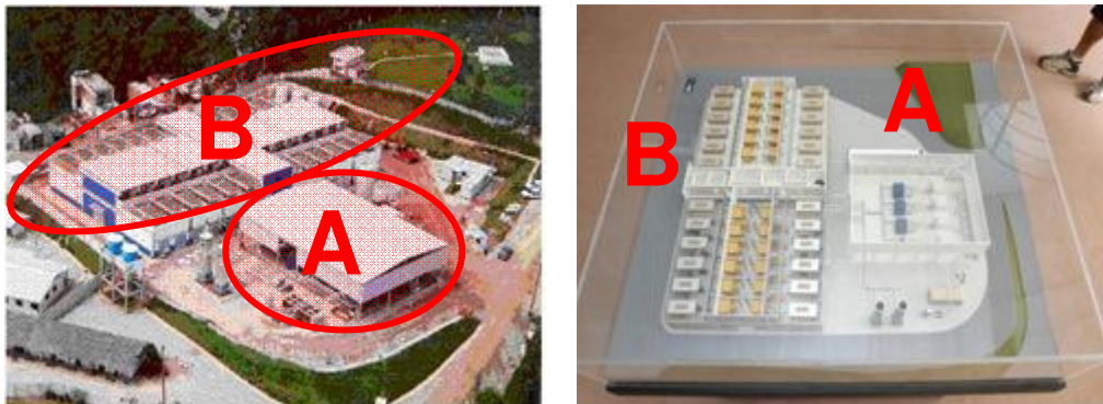
Figure 1.2. Degassing Station (A) and Power Plant (B)
