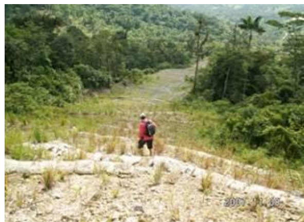
Picture 6: Revegetation of ROW of the pipe pressure
