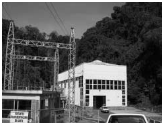
Figure 2. El Canadá power house and substation.
