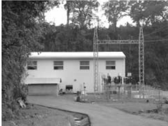
Figure 1. Montecristo power house and substation.
