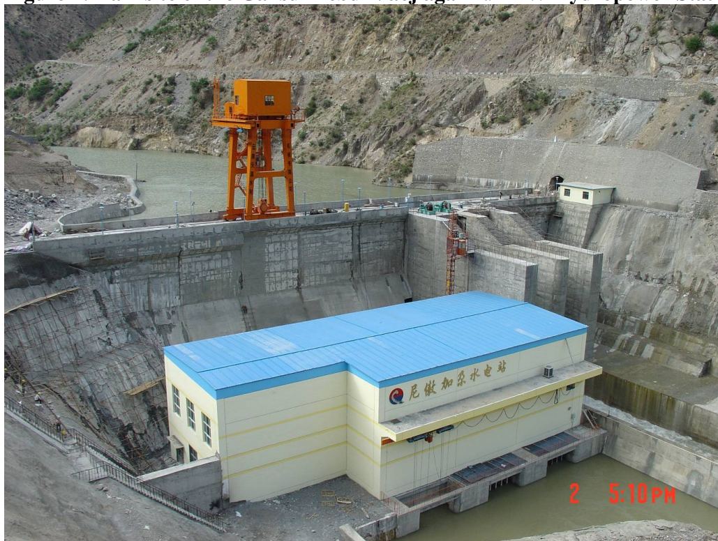
Figure 1: Dam site of the Gansu Diebu Niaojiaga 12.9 MW Hydropower Station
